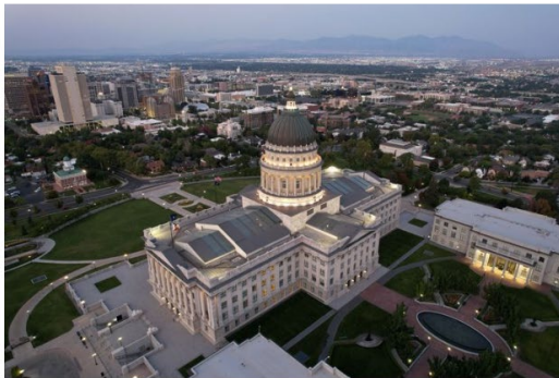
The Utah State Capitol building in Salt Lake City, Sept. 5, 2021. PHOTO: IMAGE OF SPORT/ZUMA PRESS
